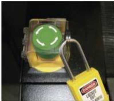
S2153 Installed Push Button and Rotary Switch Cover
